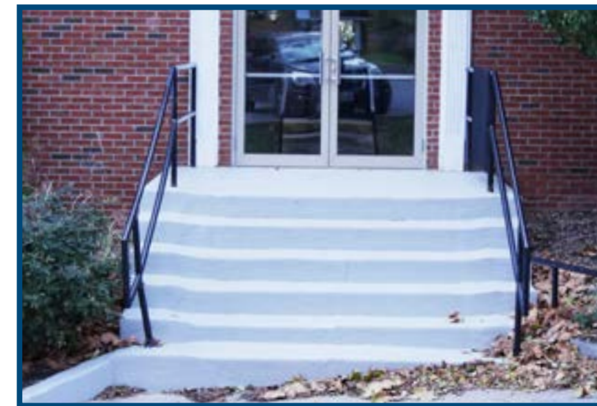
Freshly repaired and painted steps outside of the Dining Hall.
